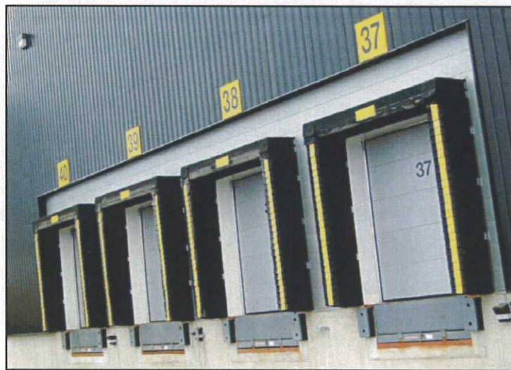
Warehouse dock doors
